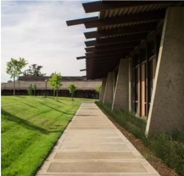
grass-lined swales are used at the base of the slope adjacent to paving
